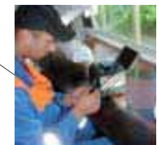
Lithuania Fiber cable welding is done in a special vehicle for getting an attenuation-free and well-functioning joint.
